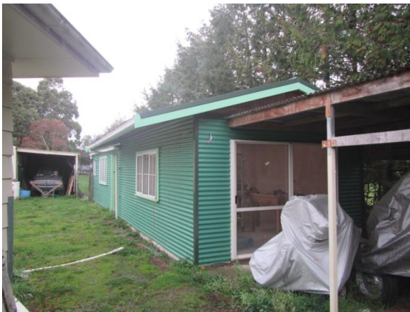
The exterior of my new office/library.
